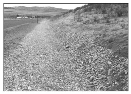
Figure 1.3. Cobble Channel Lining
