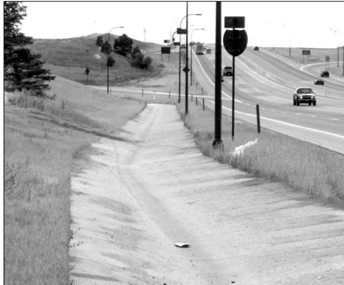
**Figure 1.1. Rigid Concrete Channel Lining**
