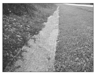
Figure 1.10. Installed Open Weave Textile Channel Lining
