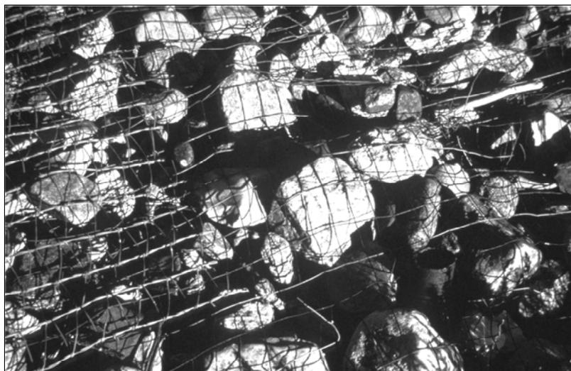
**Figure 1.5. Wire-Enclosed Riprap**
