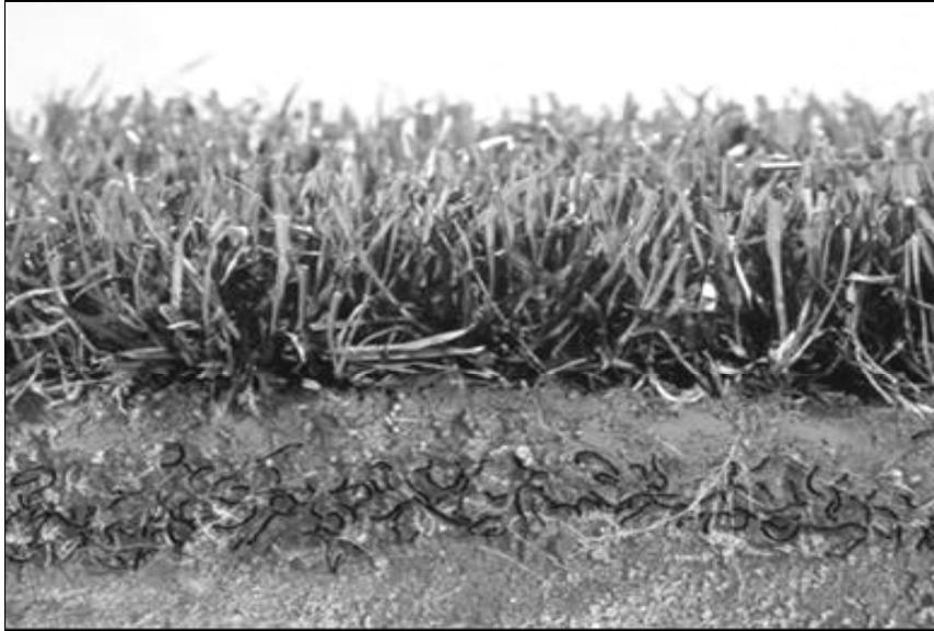
**Figure 1.7. TRM Profile with Vegetation/Soil/TRM Matrix (Source: ECTC)**
