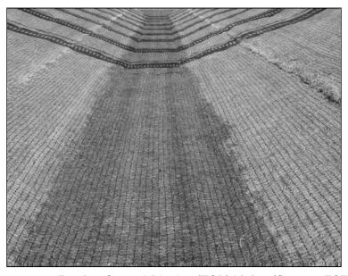
Figure 1.11. Erosion Control Blanket (ECB) Lining (Source: ECTC)
