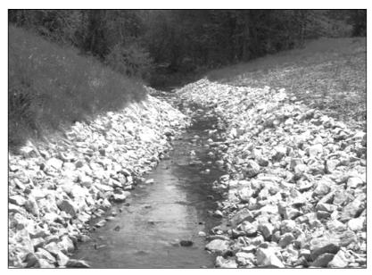
Figure 1.4. Riprap Channel Lining
