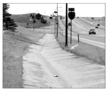
Figure 1.1. Rigid Concrete Channel Lining
