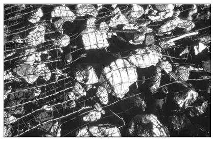
Figure 1.5. Wire-Enclosed Riprap
