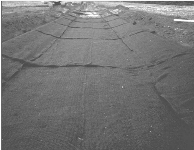
**Figure 1.8. Installed TRM Lining Before Vegetation (Source: ECTC)**
