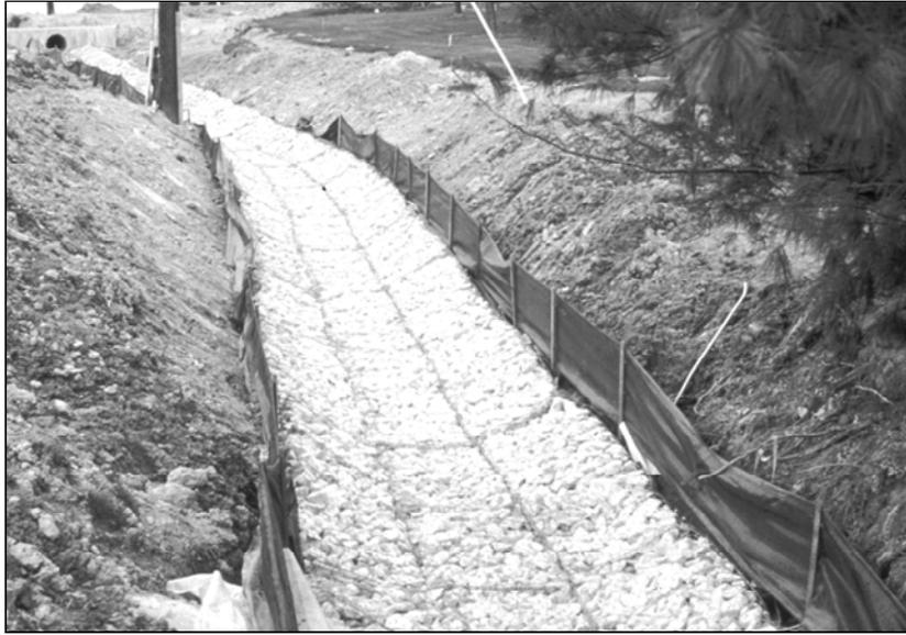
**Figure 1.6. Installed Wire-Enclosed Riprap**
