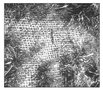
Figure 1.9. Open Weave Textile Lining
