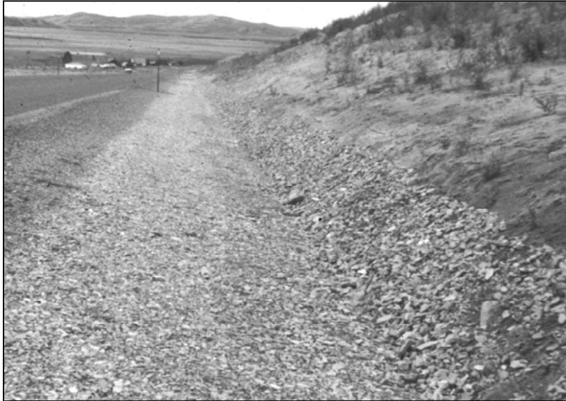
**Figure 1.3. Cobble Channel Lining**
