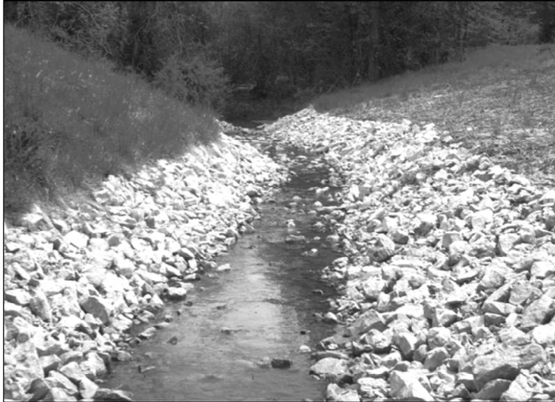
**Figure 1.4. Riprap Channel Lining**
