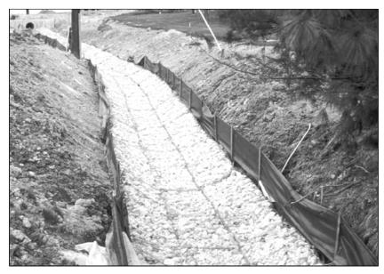
Figure 1.6. Installed Wire-Enclosed Riprap
